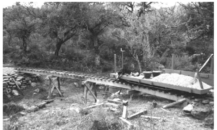
Curved trestle near completion in May 1996
