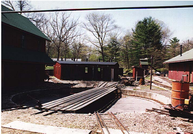
This 30' turntable serves a 5 stall roundhouse. The machine shop is at right. To the left of the turntable is where the boiler shop caught fire. In the distance between the roundhouse and the machine shop, the small green roof marks the scale coaling tower. Photo:
