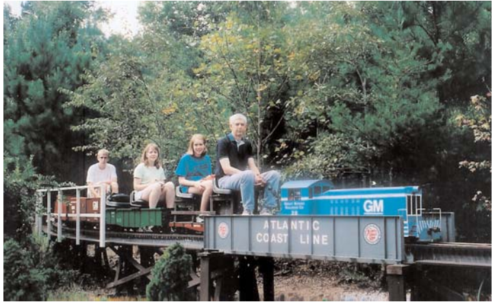
Above and below: The completed through plate girder bridge
